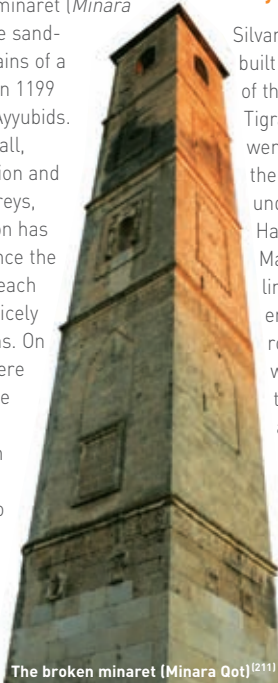
The broken minaret (Minara Qot) [211]
